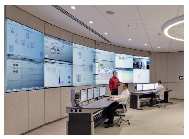
Remote Operations functionality connects multiple production facilities to a central control room with secure network technologies. It is based on standard DeltaV hardware solutions integrated into the corporate infrastructure to bring the same local user environment to the remote operators. It is an integral part of the overall iOPs solution from Emerson.
